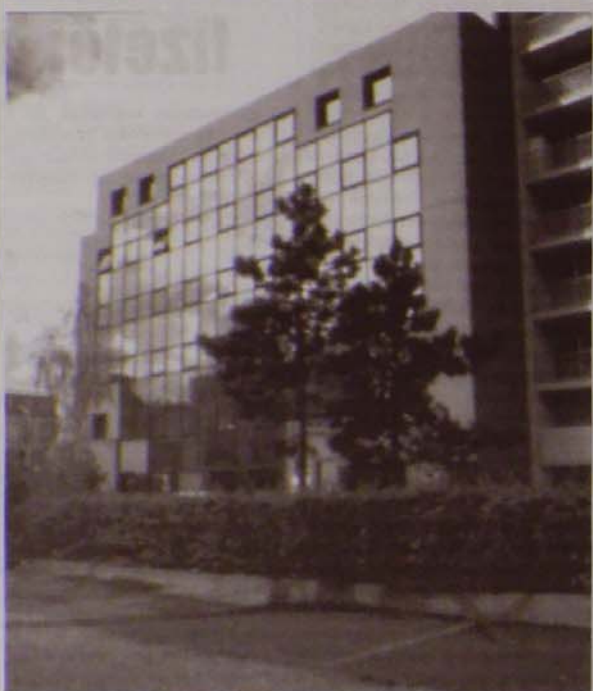
A France Telecom
